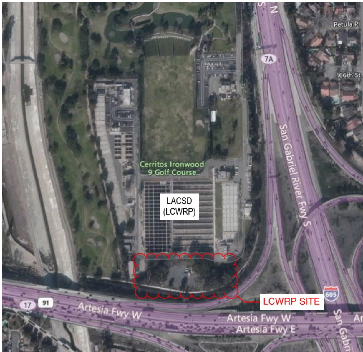
Figure 10. Los Coyotes Water Reclamation Plant Site Source: Americas Imagery Catalog (Jacobs.com)
